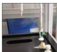
Drip cup, water faucet type and location
