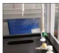
Drip cup, water faucet type and location
