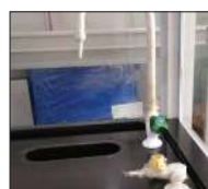
Drip cup, water faucet type and location
