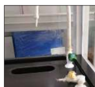
Drip cup, water faucet type and location
